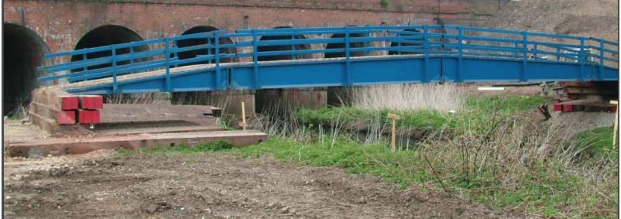
FIGURE 7 - TYPICAL TEMPORARY HGV BRIDGE
